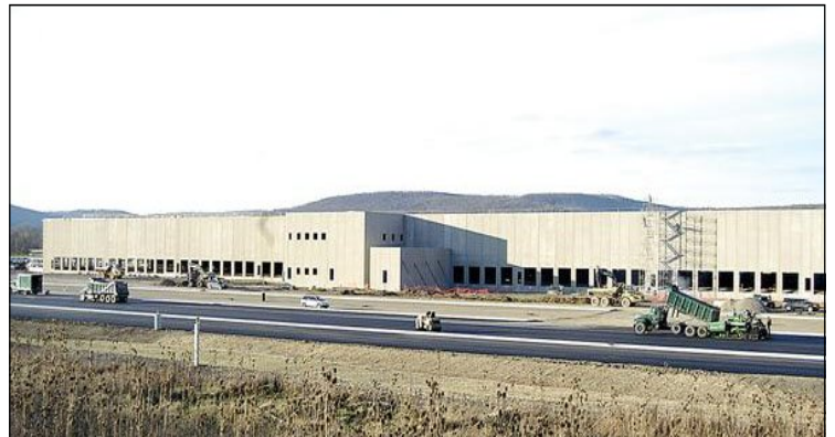
CVS Pharmacy Distribution Center under construction in the Town of Chemung.
