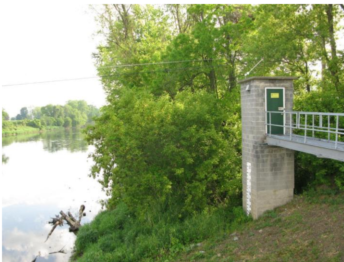
River gauge used for dam operations, levee operations, river forecasts, and other purposes.
