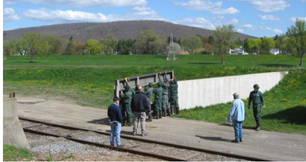
Installation of a levee closure structure.
